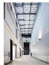
● Water Discharge Passage (55m)
