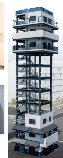
33m (11-story) Training tower
